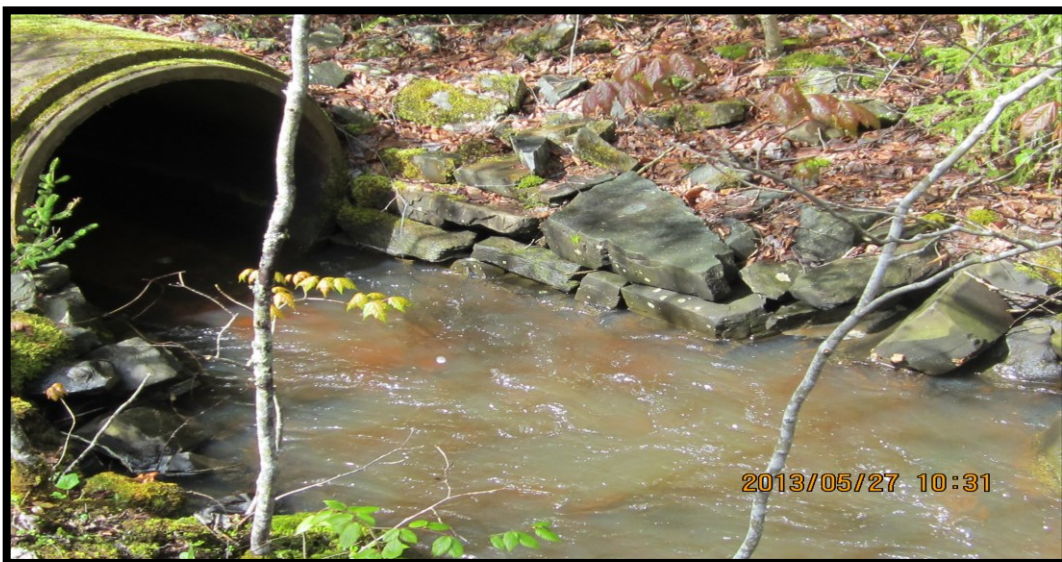
FIGURE B-2 LAGOON DISCHARGE INTO THE NATURAL WETLANDS DURING A BACKWASH EVENT
