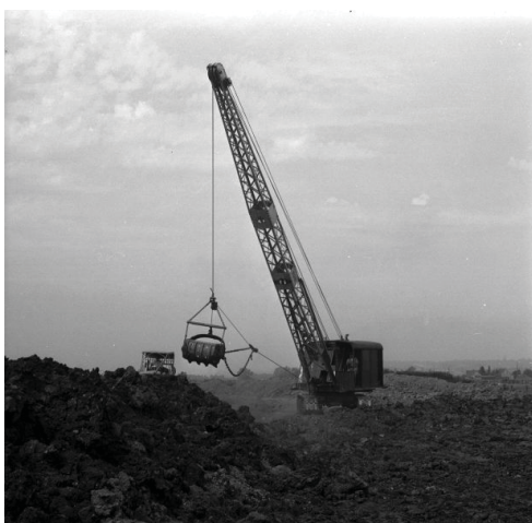
Dragline working on Serpentine and Nicolmekl rivers. (City of Surrey 2013 a)
