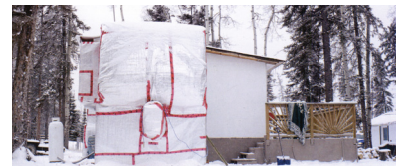
Image of mobile trailer with additional insulation and concrete addition (Hirmer 2012)
