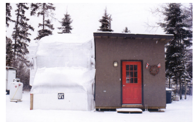
Image of trailer and addition on casters (Hirmer 2012)
