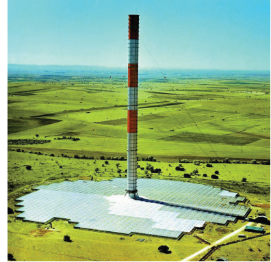
Schlaich's Solar Updraft Tower prototype in Manzanares, Spain (Meteorological Reactors 2013)
