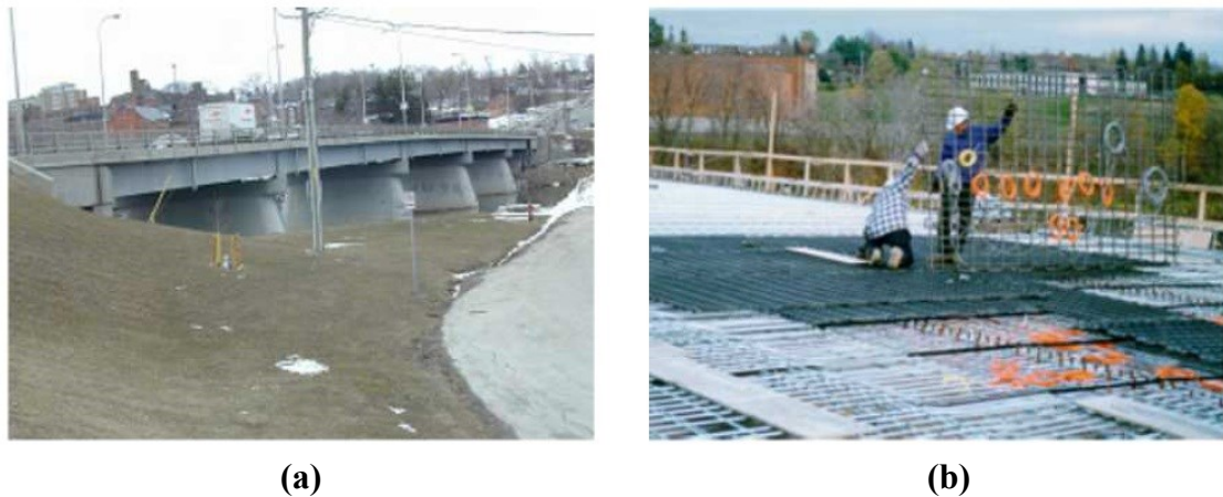
Figure 2.5 - Joffre Bridge: (a) After construction; and (b) CFRP grids (Benmokrane et al. , 2004)
