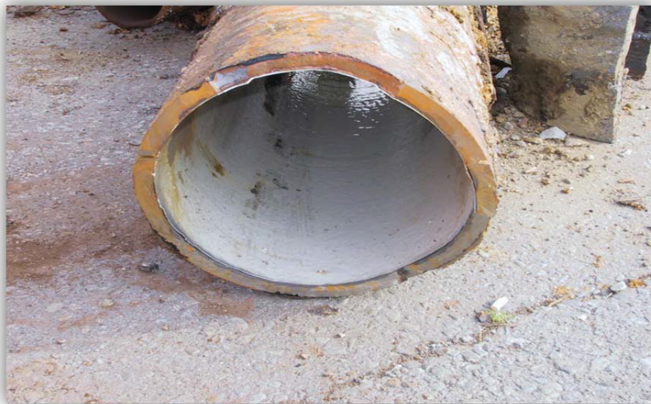
Figure 2.4 Excavated water main showing epoxy lining (Courtesy of Halifax Water).
