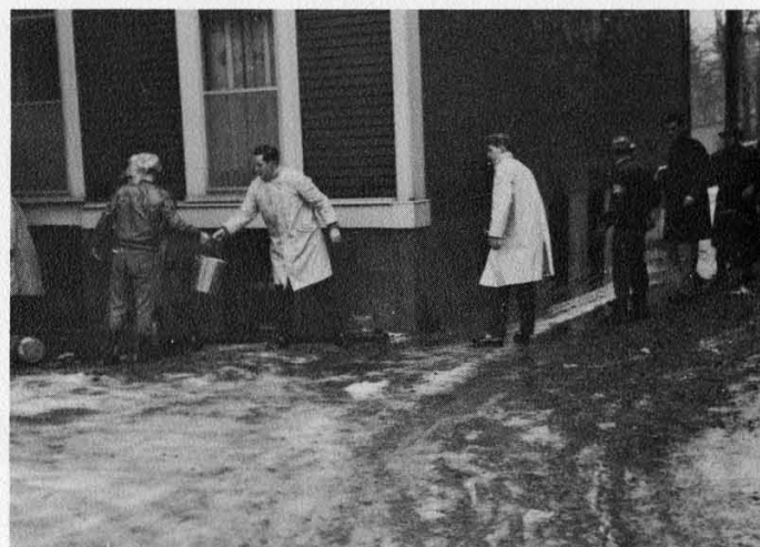
The basement was flooded. With water?
