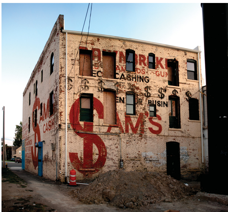
Abandoned building on Michigan Avenue, 2011.
