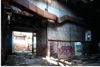
Interior of former chipping room , Detroit Dry Dock Building, 2011.
