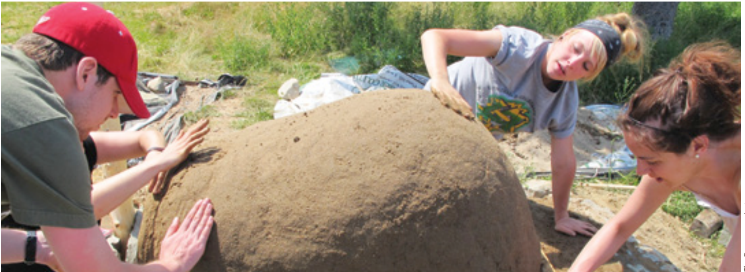
Making the sand form for the outdoor wood-fired cob oven
