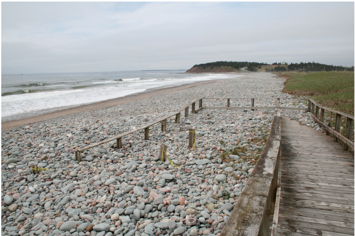
Figure 6. Storm induced damage in Lawrencetown Beach Provincial Park.
