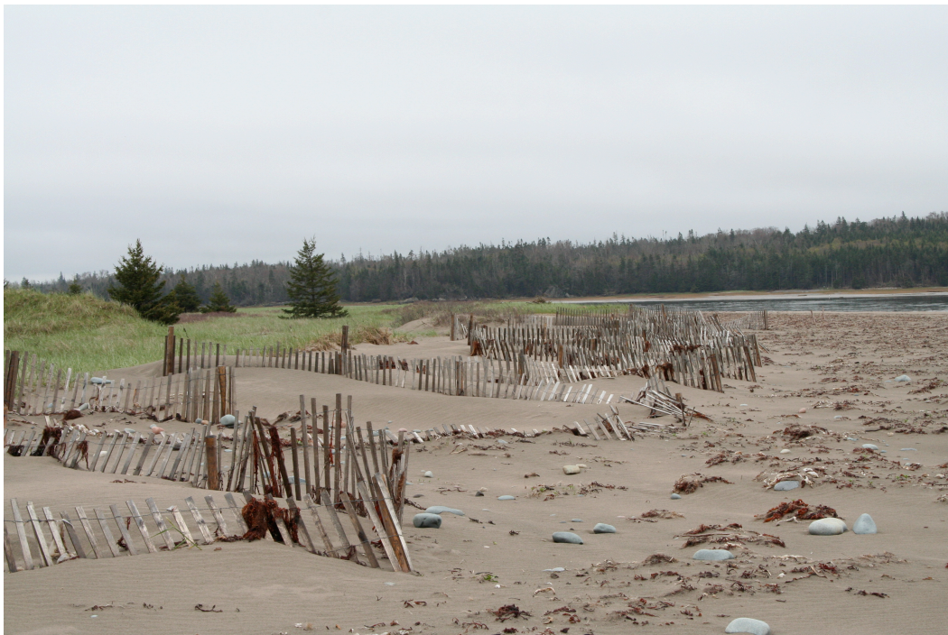
Figure 5. Dilapidated sand fences at Rainbow Haven Provincial Park.
