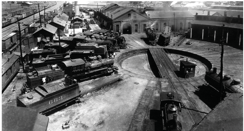
Train repair roundhouse with turntable. (Melby 2010)
