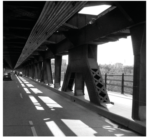
Road platform inside truss.
