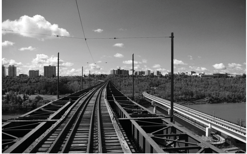
Train platform on top of truss.
