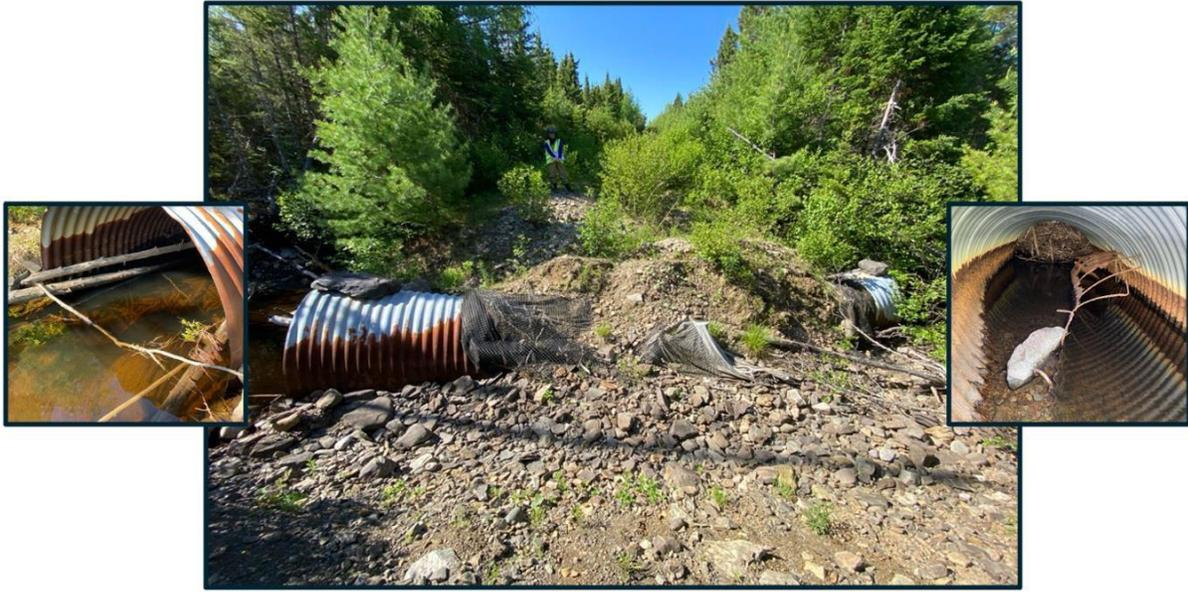
Figure 5.1 Debris clogged culvert causing road washout
