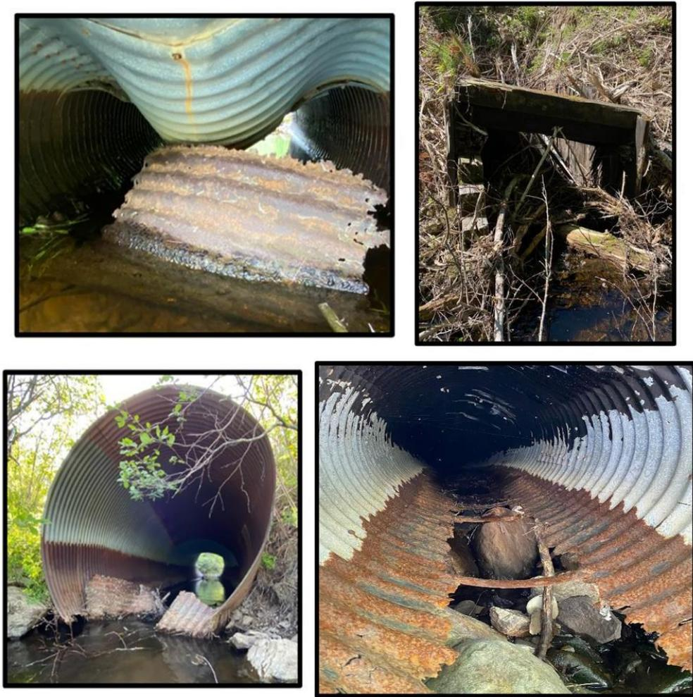
Figure 4.2 Severely deteriorated culverts in Napu'saqnuk
