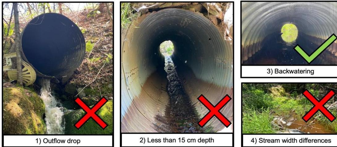
Figure 3.3 Culverts corresponding to rapid assessment criteria
