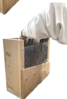
Process of stuffing eelgrass insulation in wall mock-up.
