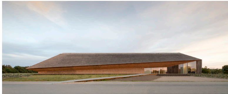
Wadden Sea Center by Dorte Mandrup, 2017 (phase 1) & 2021 (phase 2), Esbjerg, Denmark; photograph by Adam Mørk (ArchDaily 2017)
