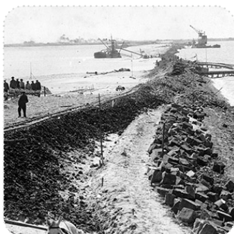
Dike construction (Reina 2021)
