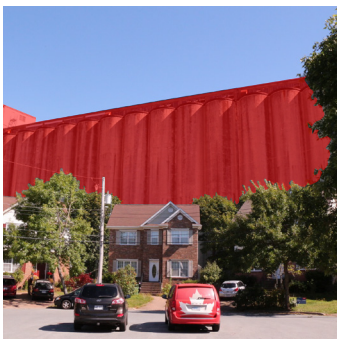
Figure 5. The height, length, and materiality of the granary make it a harsh physical barrier, evident here as it sits behind a residential area.
