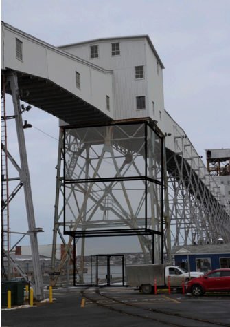
Figure 60. The seafarers tower will be contained within the existing structure of the conveyor.
