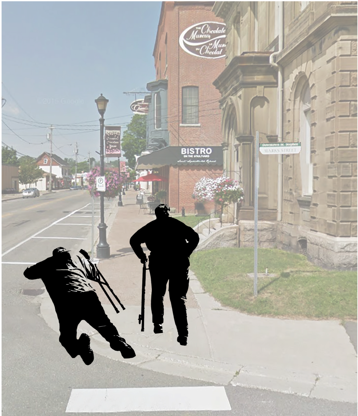
Figure 30. Frost Heave and Cracking sidewalk surfaces, St. Stephen NB, Causing an elderly man to fall into the street
