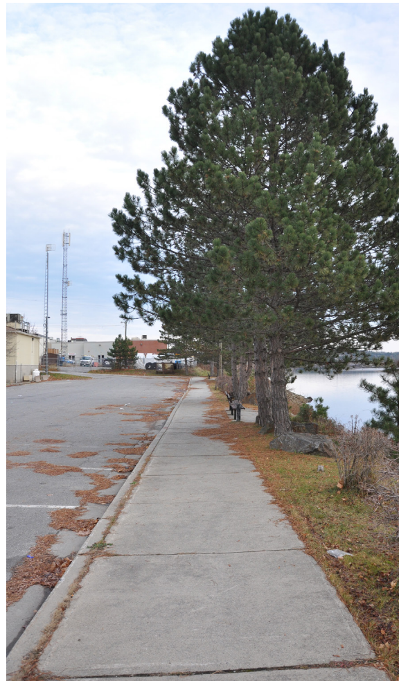
Figure 40. Uneven pavement surfaces and lack of supporting handrails for senior population; downtown St. Stephen NB, along the St. Croix River
