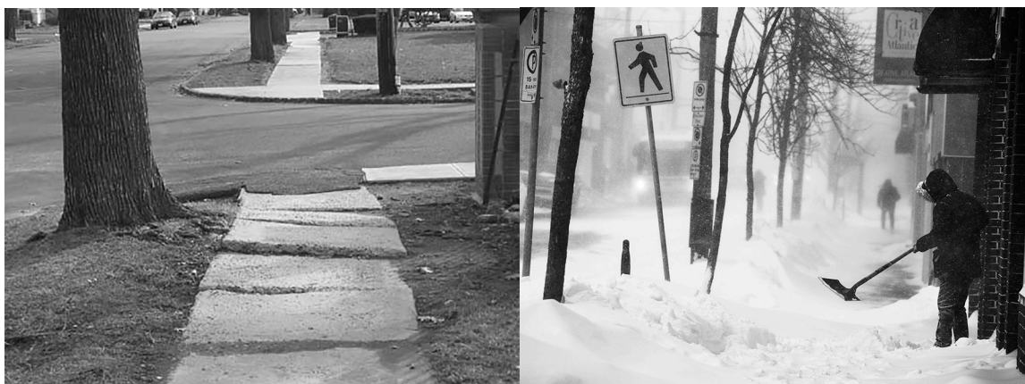
Figure 29. Frost Heave and Cracking sidewalk surfaces in St. Andrews, NB alongside image of winter storm in Halifax, NS. Hazardous Circulation routes for seniors; photographs by author
