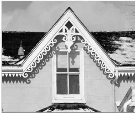
FIG. 13. DORMER OF NEWLANDS'S 1883 ADDITION. | JENNIFER MCKENDRY.
