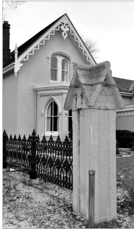
FIG. 16. STONE PIER BY EDWARD HORSEY, 1862, AND CAST-IRON FENCE BY WILLIAM NEWLANDS, 1883. | JENNIFER MCKENDRY.
