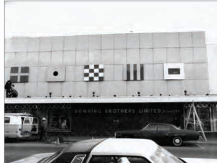
FIG. 12. BOWRING BROTHERS STORE. VIEW OF THE ORIGINAL STOREFRONT FACING WATER STREET, WITH CONTINUOUS PLATE GLASS DISPLAY WINDOWS AND CANTILEVERED CANOPY, 1970S. | ST. JOHN'S CITY ARCHIVE, 26-01-025.
