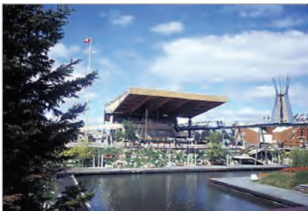
FIG. 23. ATLANTIC PROVINCES PAVILION, EXPO 67, 1967, ÎLE NOTRE-DAME, MONTREAL, QC (DEMOLISHED). ARCHITECTURAL FIRM: DUFFUS ROMANS SINGLE AND KUNDZINS, HALIFAX. DESIGN CONSULTANTS: PROF. OJARS BISKAPS AND PROF. DOUGLAS SHADBOLT, SCHOOL OF ARCHITECTURE, NOVA SCOTIA TECHNICAL COLLEGE, HALIFAX. GENERAL VIEW SHOWING BLACK SPRUCE ROOF CANOPY AND CONCRETE RAMPS, WITH THE MONORAIL TRACK AT RIGHT, 1967. | PHOTOGRAPH: ERNEST MAUNDER. LIBRARY AND ARCHIVES CANADA.
