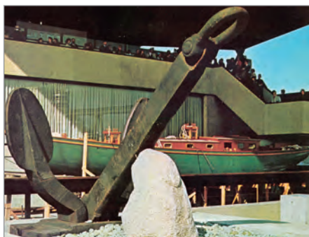
FIG. 25. ATLANTIC PROVINCES PAVILION, EXPO 67. VIEW OF ATLANTICA UNDER CONSTRUCTION IN THE BOATYARD UNDER THE CANOPY, WITH THE VIEWING GALLERY BEHIND, 1967. | PHOTOGRAPH: FROM DE LORIMIER, EXPO 67 - MONTREAL, CANADA, P. 133.
