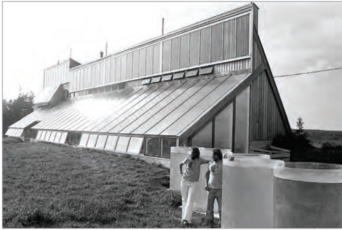
FIG. 16. THE PEI ARK, 1975-1976, SPRY POINT, LITTLE POND, PE (DEMOLISHED). ARCHITECTURAL FIRM: SOLSEARCH ARCHITECTURE, CHARLOTTETOWN, PE, AND CAMBRIDGE, MA. DESIGN ARCHITECTS: DAVID BERGMARK AND OLE HAMMARLUND. DAVID BERGMARK AND OLE HAMMARLUND IN FRONT OF THE SOUTH WALL AND SOLAR COLLECTOR PANELS, N.D. | BERGMARK HAMMARLUND JONES COLLECTION.
