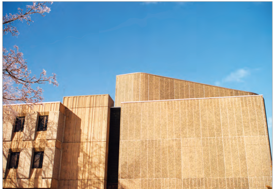
FIG. 3. DALHOUSIE ARTS CENTRE, DALHOUSIE UNIVERSITY, 1969-1971, HALIFAX, NS. ARCHITECTURAL FIRM: C.A. FOWLER BAULD AND MITCHELL LTD., HALIFAX, NS. DESIGN ARCHITECTS: CHARLES A. FOWLER, ANDREW LYNCH, JUNJI MIKAWA. DETAIL OF PRECAST CONCRETE CLADDING AND CONCRETE STRUCTURE, MAY 2001. | CHAD JAMIESON.
