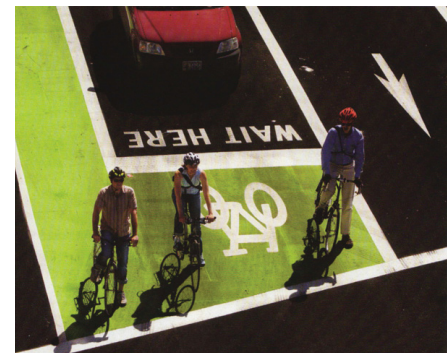
Integration of infrastructure supports co-existence of bicycles and vehicles, Portland (Land 8 2013)
