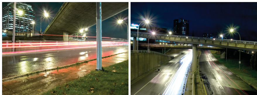
Night views of Cogswell Interchange - motion and light
