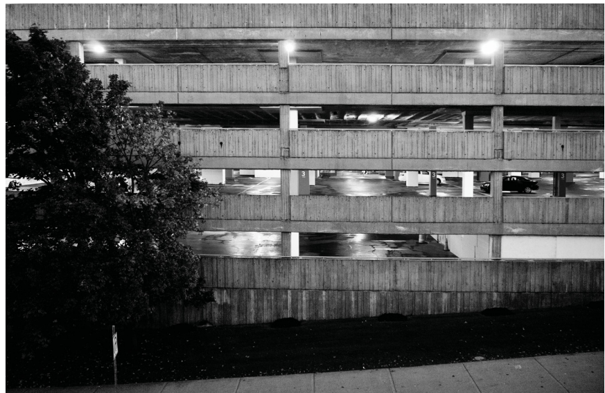
Parking structure at Cogswell Street
