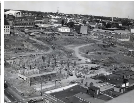
Duke St construction, 1967 (Nova Scotia 2013)
