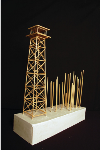
Fire Tower case study showing a 90' tower with small open cab.
