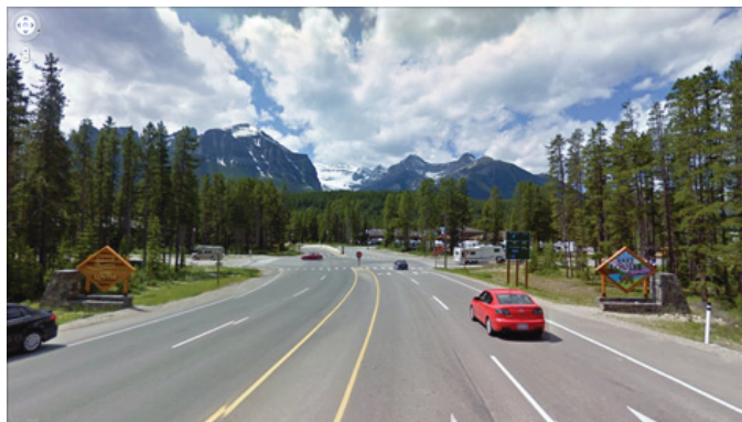
Figure 11 Image of entrance to town from the Trans Canada Highway. Lake Louise Drive dominates the crossroads and encourages traffic to continue ahead instead of turning onto Village Road and into town. (Google Maps, accessed 4 January 2011)
