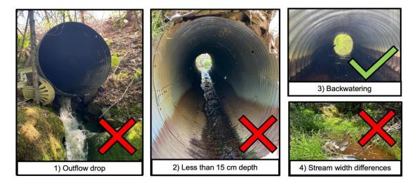
Figure 3.3 Culverts corresponding to rapid assessment criteria
