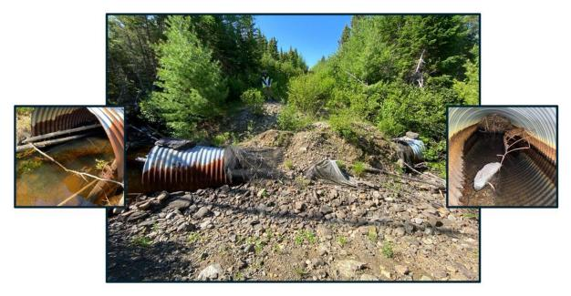
Figure 5.1 Debris clogged culvert causing road washout
