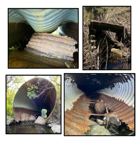
Figure 4.2 Severely deteriorated culverts in Napu'saqnuk
