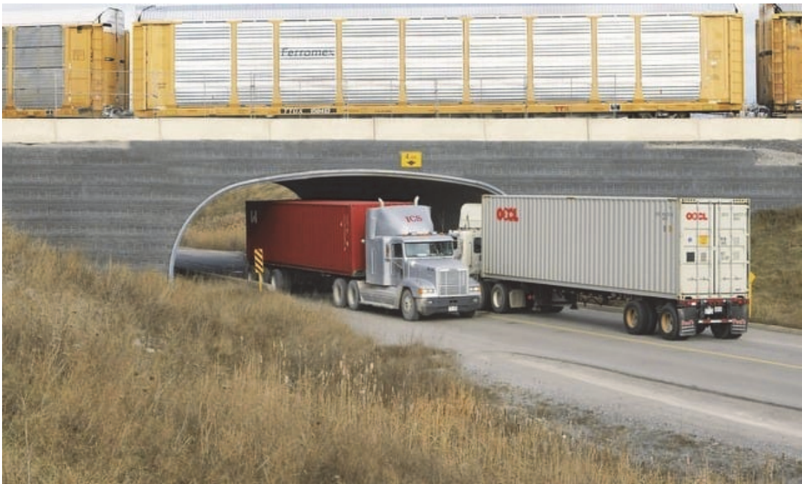
Figure 1.1. An example of a Corrugated Box Culvert used for highways and railways (Atlantic Industries Limited)
