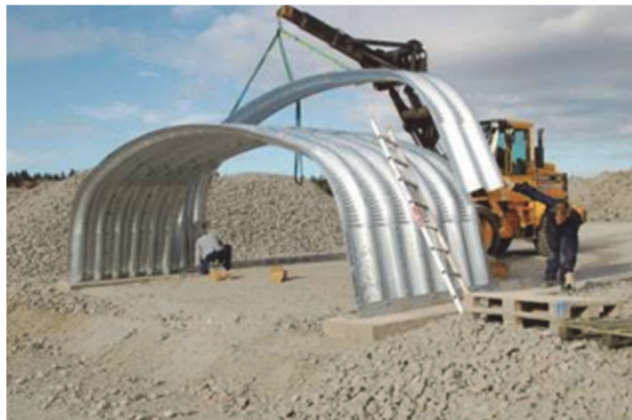
Figure 3.1 A corrugated box culvert profile under construction (Sweden 2006).
