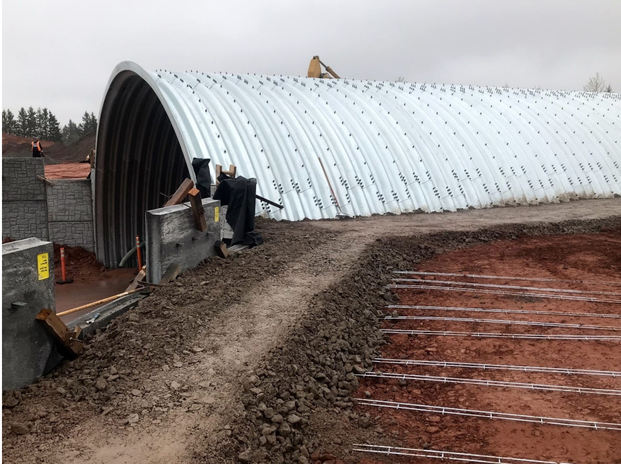
Figure 1.1 Baltic Road Arch at Trans Canada Highway, Clyde River, PEI
