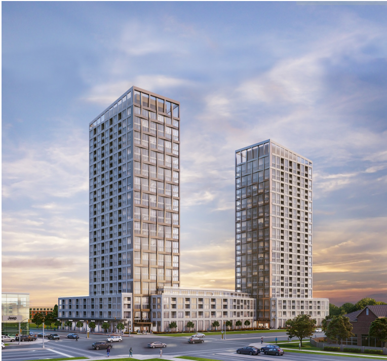
Figure 67. SmartCentres Oakville North, a high-density, mixed-use development at the corner of Oak Park and Trafalgar, reflecting the incentives of the main street and the future bus lane, rather than the car-oriented arterial and the car-dealership across the road (Source: Landau 2021).
