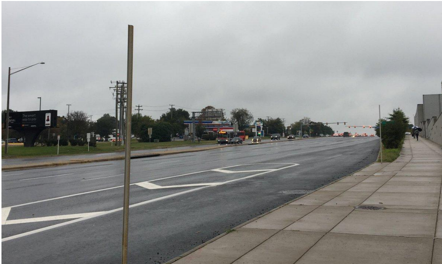
Figure 52. The results of a recent sidewalk improvement on Route 123. (Source: photo by Stewart Schwartz, used with permission.)
