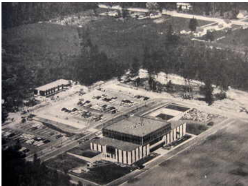
Figure 36. 1962 Surrey City Hall (Source: Brown 2014c).
