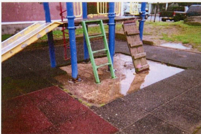
Dangerous Playground in Greystone Public Housing Area. Photographed by Tracey.
