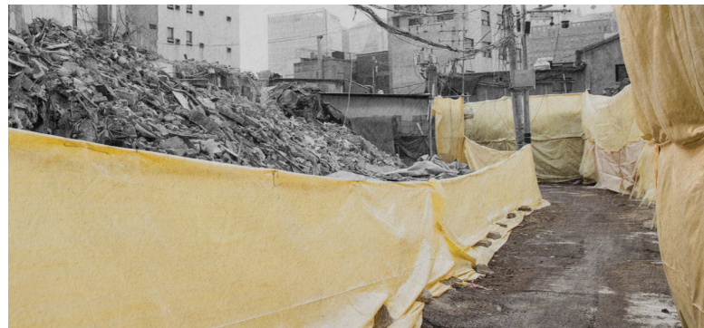
Demolition happening in Euljiro (Listen to the City 2019)
