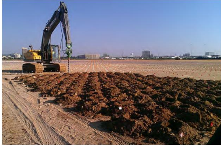
Figure 2.16: PVD's installed at 0.9m at the Gulfport site (Goldberg 2013)
