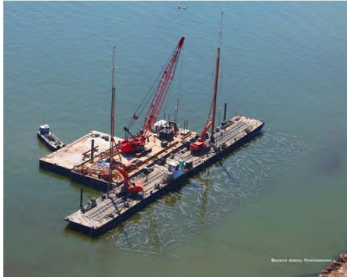
Figure 2.14: PVD installation at the site (Goldberg 2013)
