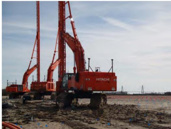
Figure 2.15: Installation of PVD at the container site (Goldberg 2013)
