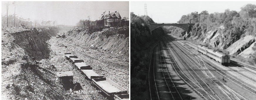
Image of the railway "cut" being blasted, and the from the same perspective 60 years later. Images: Nova Scotia Archives
