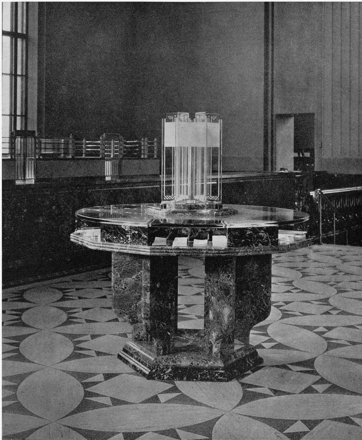
CHEQUE DESK IN MAIN BANKING ROOM, BANK OF MONTREAL—OTTAWA
