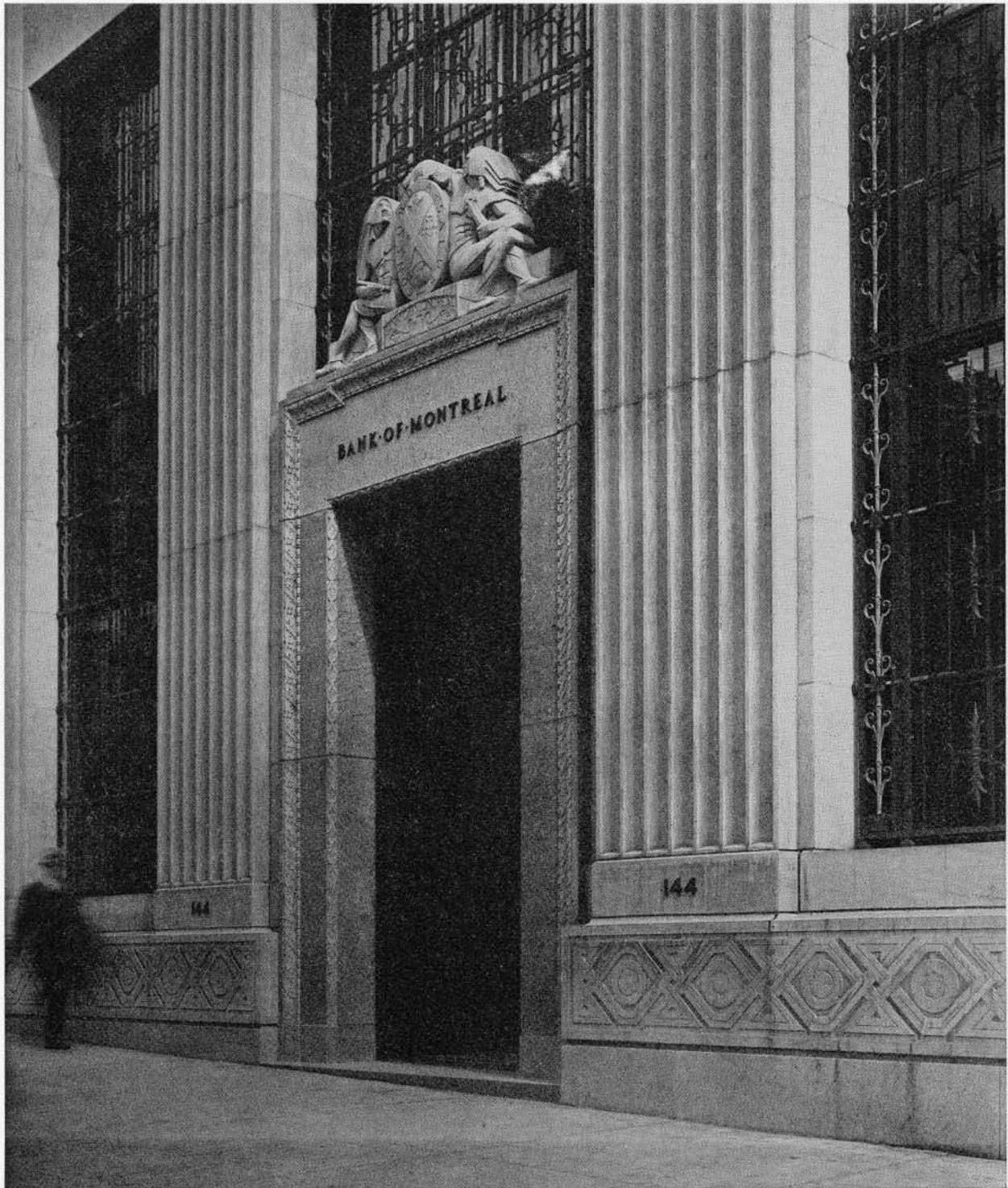
DETAIL OF NORTH ENTRANCE BANK OF MONTREAL BUILDING, OTTAWA Barott & Blackader, Architects
