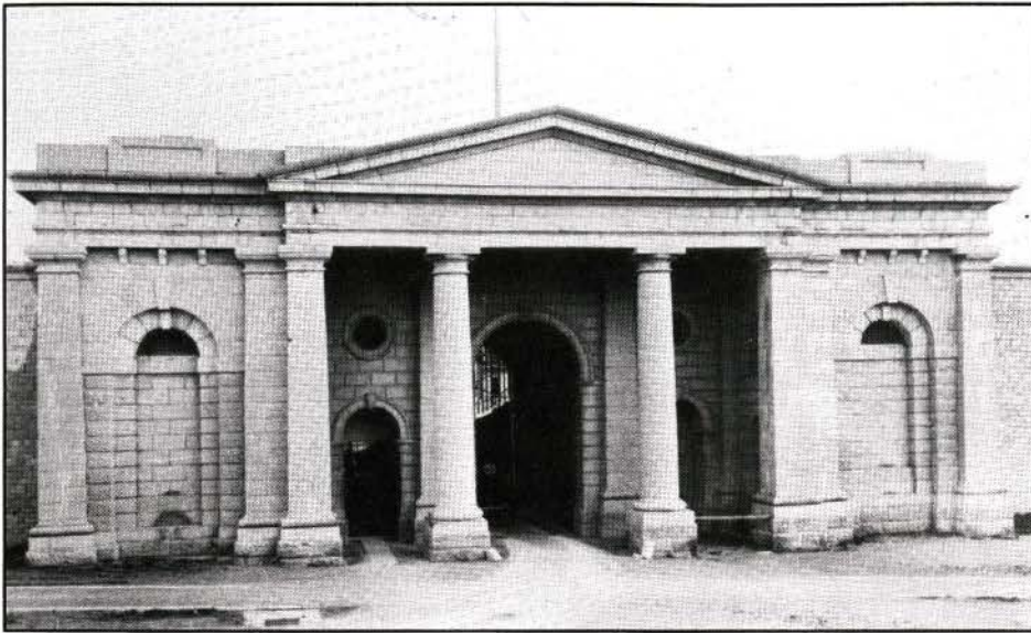
Figure 6. William Coverdale, Provincial Penitentiary, 1840-44, exterior of north gateway before the addition of a central tower about 1895. (Queen's University Archives)
