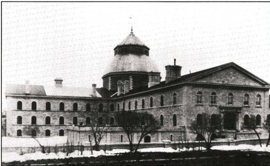
Figure 4. William Coverdale and Edward Horsey, Provincial Penitentiary, beg. 1833, north-east view of Main Building before the alterations of the windows and doorway in the early 20th century. (Queen's University Archives)
