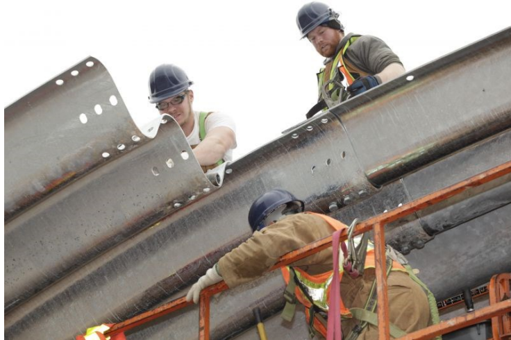
Figure 4-9: Crew securing longitudinal joint.
