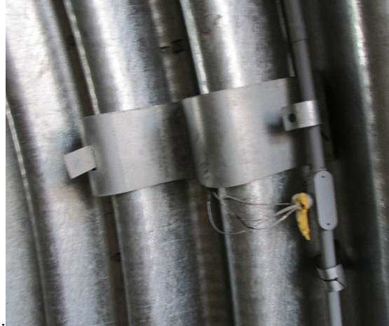
Figure 4-19: Protection steel plate
