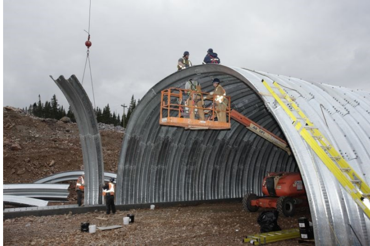
Figure 4-7: Side component assembly on the Corner Brook structure
