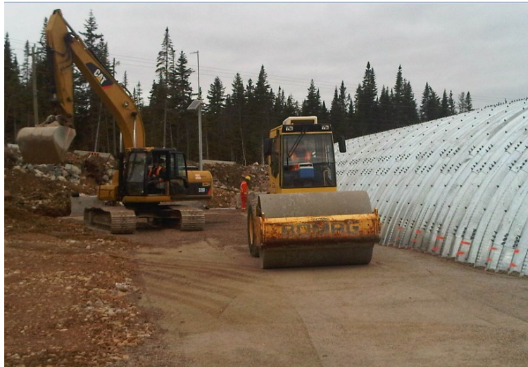
Figure 4-11: Compaction of backfill, Corner Brook
