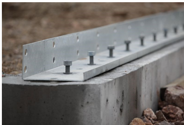
Figure 4-4: Base channel on the Corner Brook structure
