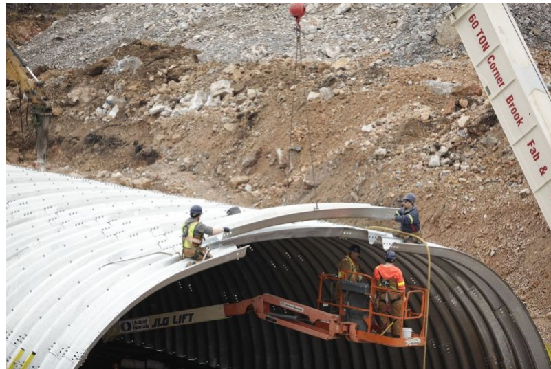
Figure 4-8: Placement of top plate
