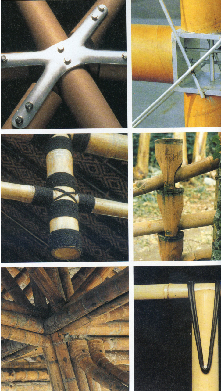
Examples of modern bamboo joinery (Kries and von Vegesack 2000, 114)
