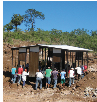
Community moving temporary house to make room for permanent construction
