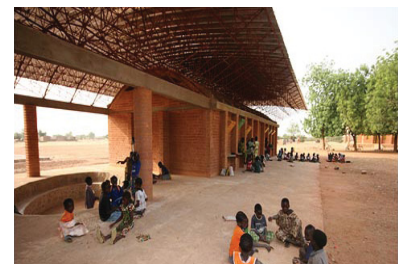
School extension, amphitheater (Kéré 1999)
