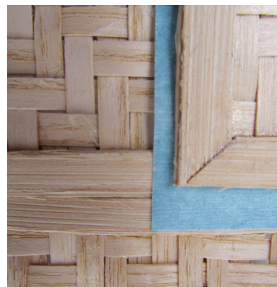
Photograph of model showing roof cladding: a layering of woven panel - tarp - woven panel. This creates a roof that is lightweight in comparison to traditional tiled roofs providing increased seismic safety. Also, this does not trap heat in the same way sheet metal roofs do (another common roofing material).
