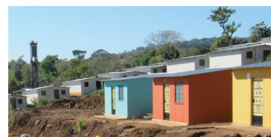
Permanent housing: hand poured concrete walls, tile floor, sheet metal roof.
