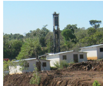
Temporary shelters: light metal frame, cardboard cladding, thin sheet metal roof, and dirt floor.
