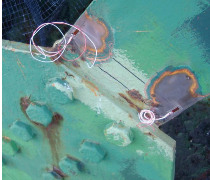
Figure 5-6 : Flange gauge pair next to diagonal gusset plate
