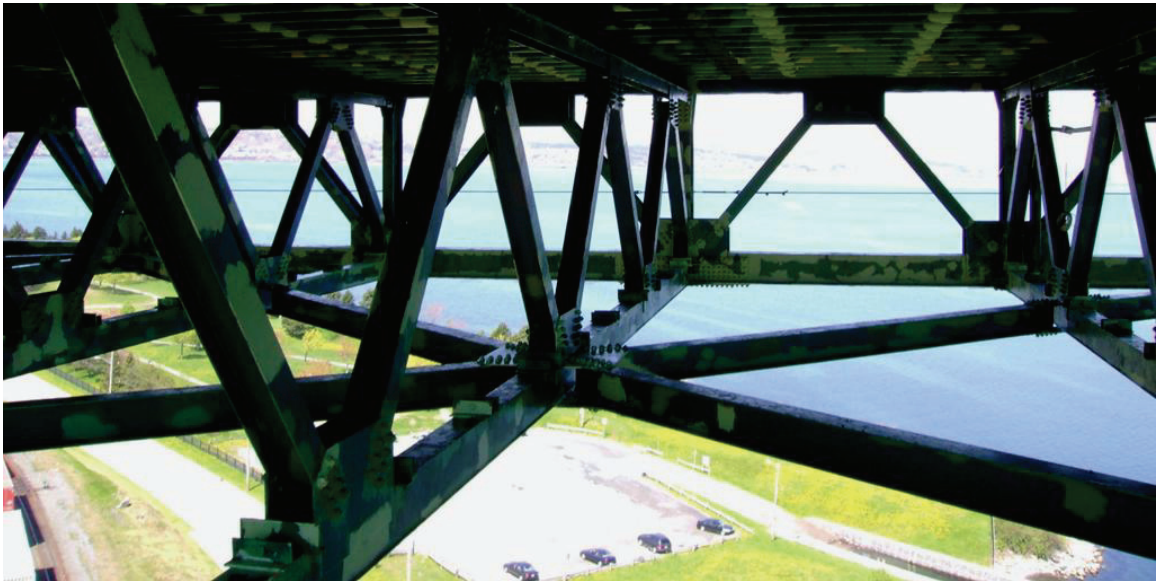
Figure 5-4 : Lateral stiffening truss
