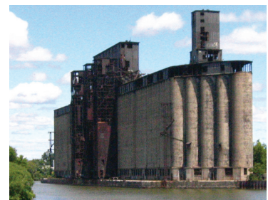
Precedents: (Top) James Stirling, Florey Hall, 1971. The Residence frames a quad. Services and circulation are attached to the form. From Seier Plus Seier. (Bottom) Marine legs attached to the side of Concrete Central grain terminal, Buffalo.
