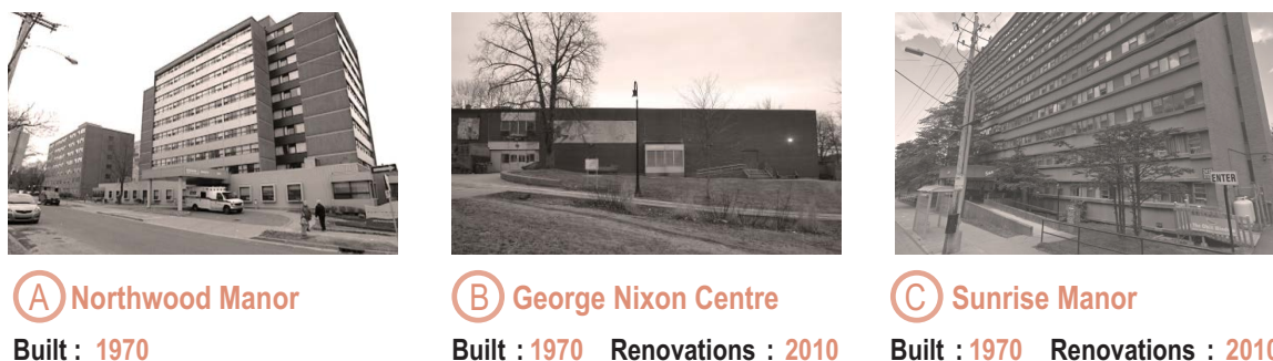
Figure 3.6 : Site Analysis of Existing Buildings
