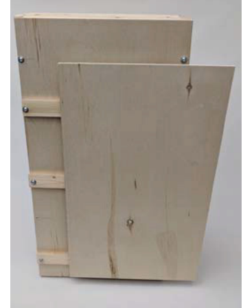
1/4 scale construction details of bolted interior wall panels and attached french cleat hangers
