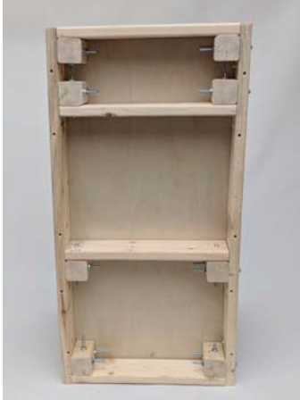
1/4 scale construction details of bolted interior wall panels and attached french cleat hangers
