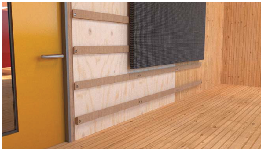
Wall panel with pin board mounted on french cleats
