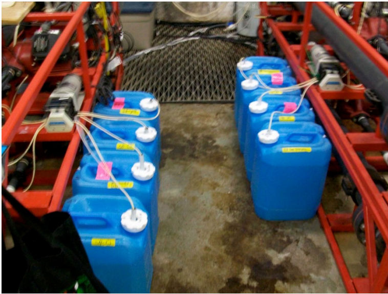
Figure 3.7 Chemical jugs set up for pipe loops
