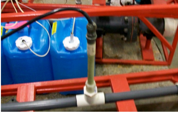
Figure 3.10 Two-electrode linear polarization probe used in pipe loop
