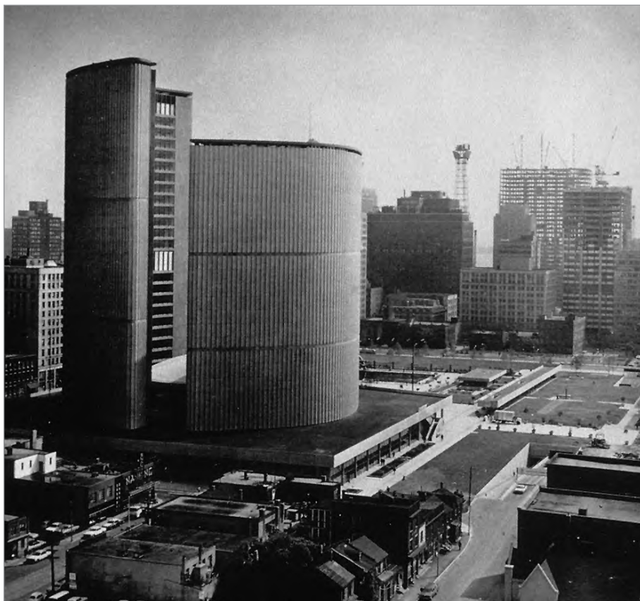
FIG. 14. VILO REVELL AND PARKIN ASSOCIATES, TORONTO CITY HALL, COMPETITION 1956-1958 AND CONSTRUCTION 1961-1965, PHOTOGRAPHED C. 1967.
