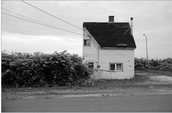
FIG. 37. "HALF DUPLEX" AFTER DEMOLITION OF ITS OTHER HALF IN GLACE BAY. | MARIANNE CHARLAND.
