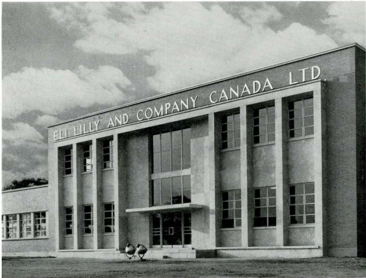
DETAIL OF MAIN ENTRANCE
