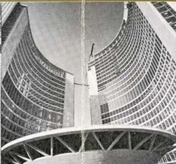
Precast struts on council chamber
