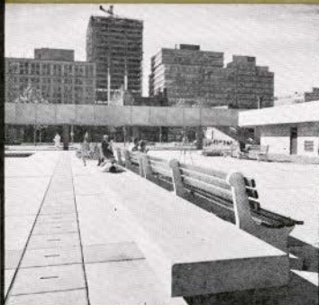
Duct covers and benches
