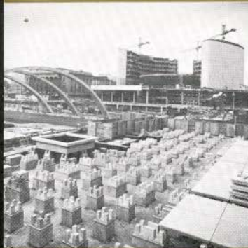
Precast pedestals supporting paving
