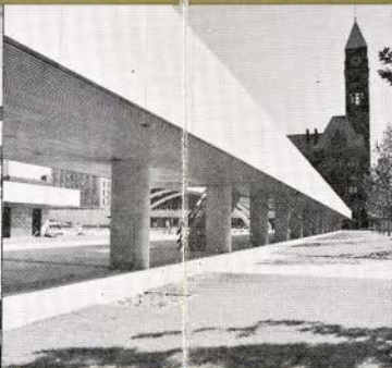
Balustrades to elevated walkway
