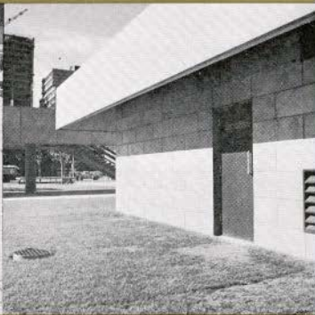
Pool house wall panels and fascia
