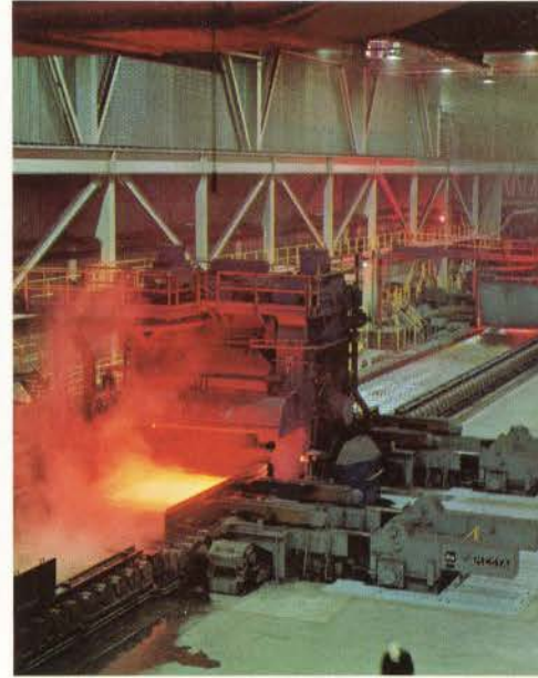
The plate mill itself—newest and widest in Canada—can produce plate in widths up to 140" and thicknesses from 3/16" to 6".
