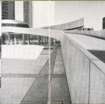
Paving and balustrade
