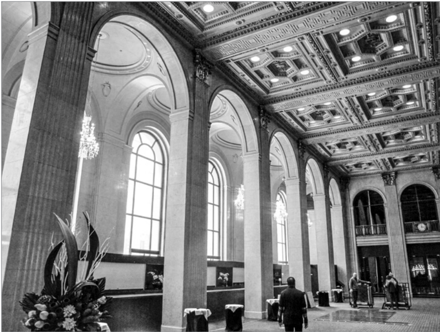
FIG. 26. DOMINION BANK MAIN HALL AND GALLERY. NOTE THE SOANIAN SHALLOW DOMES. | DAVID E. WINTERTON, 2015.
