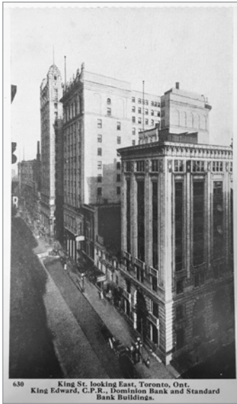
FIG. 22. VIEW LOOKING EAST ALONG KING STREET WEST: A SHOWCASE OF DARLING AND PEARSON'S TERRACOTTA PORTFOLIO ON BANKERS ROW: THE COMMERCE BANK, THE DOMINION BANK, AND CPR BUILDING. POSTCARD, AFTER 1918. | TORONTO ARCHIVES.
