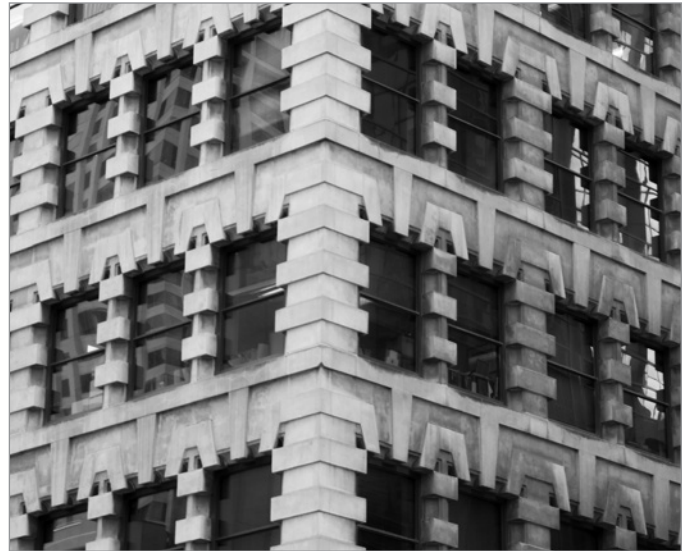
FIG. 16. THE LUMSDEN BUILDING'S GIBBS SURROUNDS, DETAIL. | DAVID E. WINTERTON, 2015.
