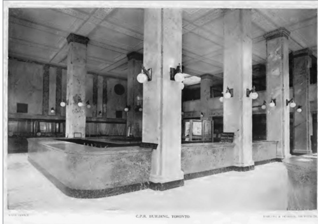
FIG. 18. CPR BUILDING GROUND FLOOR INTERIOR. | CONSTRUCTION, 1913, VOL. 4, NO. 8, P. 293.
