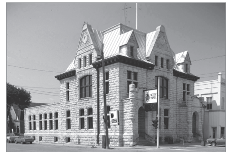
FIG. 10. POST OFFICE, PORTAGE-LA-PRAIRIE, MANITOBA; BUILT 1896-1899. | PARKS CANADA, HERITAGE RECORDING SERVICE, 252, 1980.
