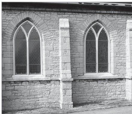
FIG. 14. BARRIEFIELD, ST. MARK'S, DETAIL OF SOUTH SIDE. | PAUL CHRISTIANSON, 2006.
