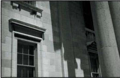
Fig. 12. First storey, side wing window with a plain frieze (window to the left). (Photo: Venetia Stewart)
