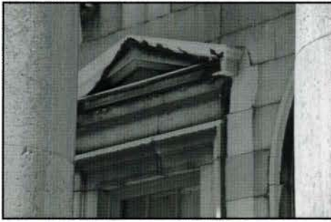
Fig. 11. First storey, centre block window with a pulvinated frieze. (Photo: Venetia Stewart)
