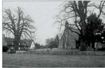
FIG. 3. LONG STANTON (CAMBRIDGESHIRE), ST. MICHAEL'S, GENERAL VIEW FROM SOUTHWEST. | MALCOLM THURLBY
