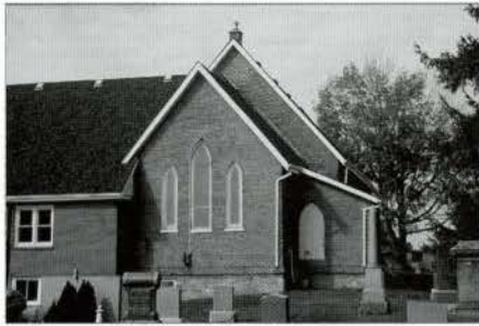
FIG. 6. GLANFORD, ST. PAUL'S, EXTERIOR FROM EAST. | MALCOLM THURLBY
