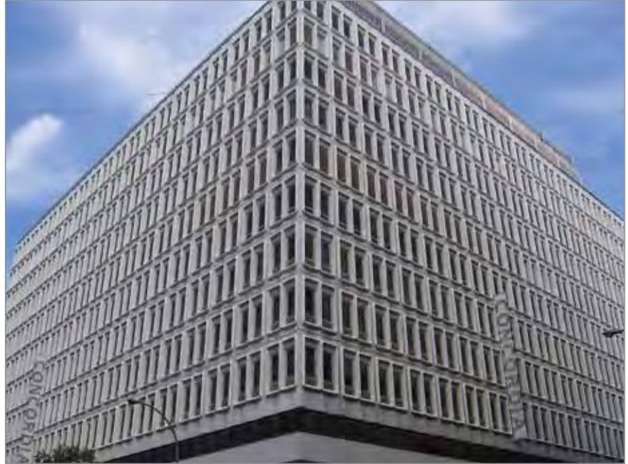
FIG. 16. PREFABRICATED CONCRETE CURTAIN WALL OF REMARKABLE ELEGANCE. | ANJA BORCK.
