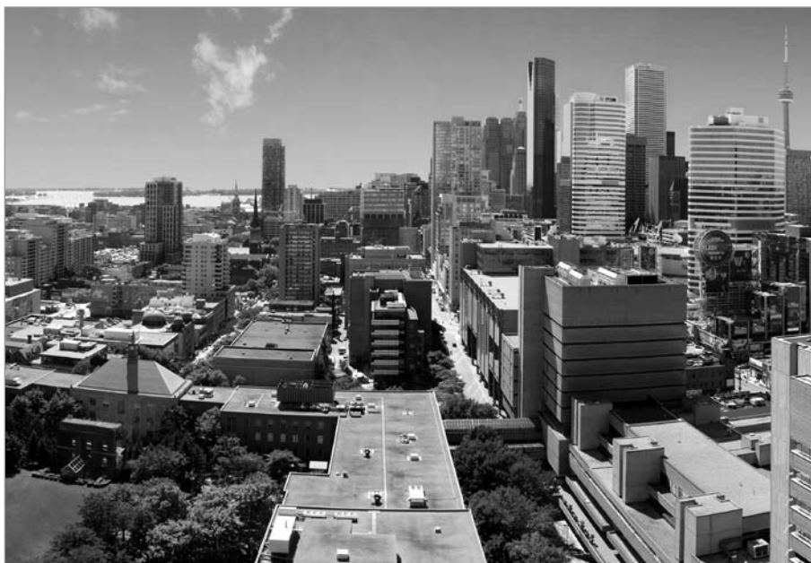
FIG. 1. RYERSON UNIVERSITY PANORAMA (DETAIL). | COURTESY OF RYERSON UNIVERSITY.
