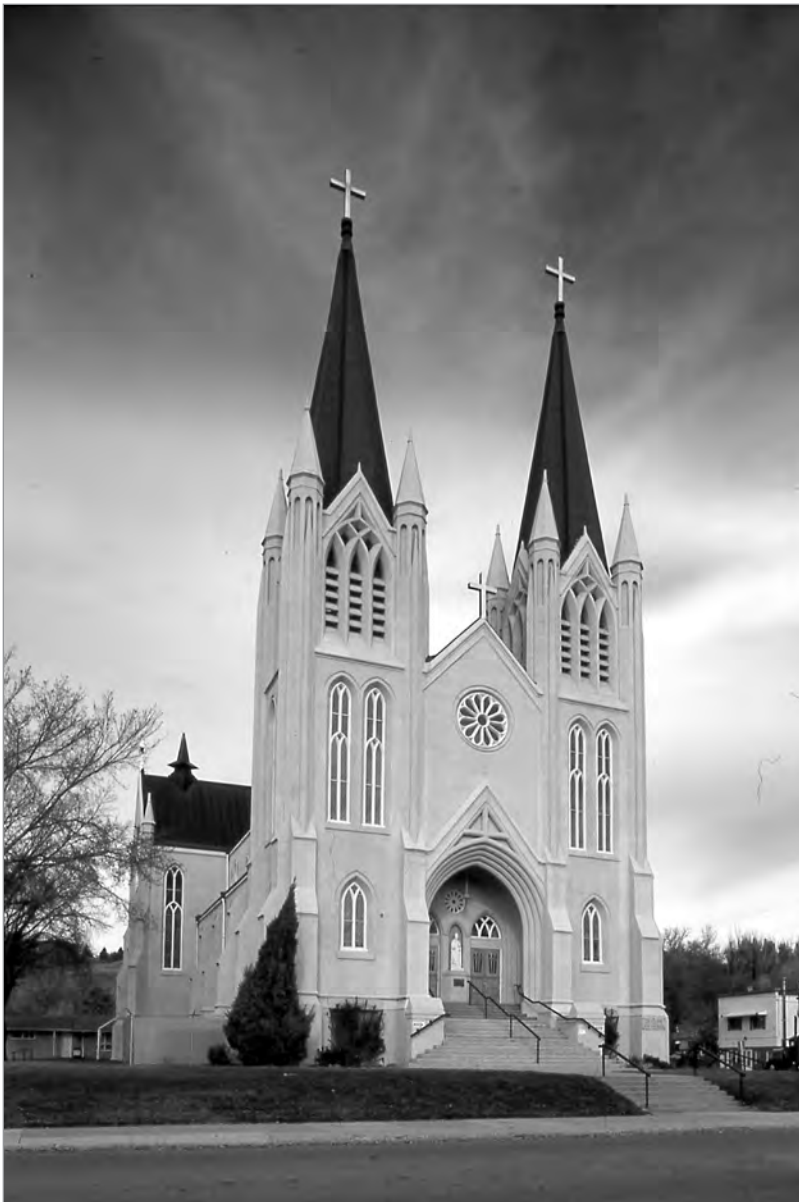
FIG. 1. VIEW OF WEST FAÇADE OF THE FIRST CHURCH IN CANADA FABRICATED FROM REINFORCED CONCRETE. ST. PATRICK'S ROMAN CATHOLIC CHURCH, MEDICINE HAT, ALTA. (1912-1914). ARCHITECT: MANLY N. CUTTER. | BARRY MAGRILL
