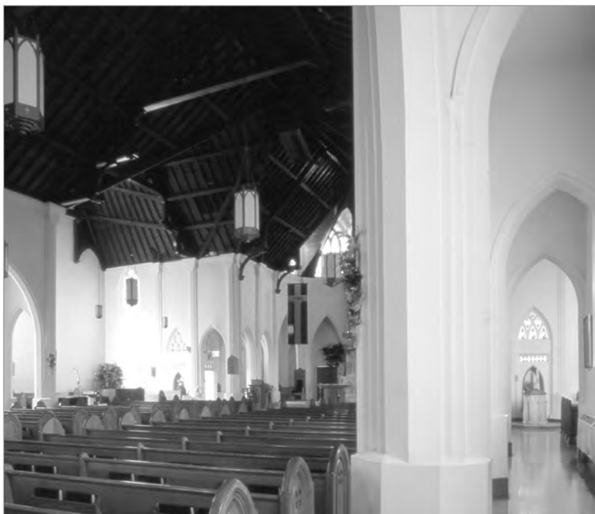
FIG. 6. VIEW OF NAVE LOOKING EAST AND INTO THE AISLE THAT SHOWS THE SIMPLE PIERFORM MOULDING. ST. PATRICK'S ROMAN CATHOLIC CHURCH, MEDICINE HAT, ALTA. (1912-1914). | BARRY MAGRILL
