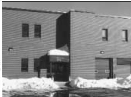
A view of the completed Aquaculture wing as seen from behind the Animal Science Building.
