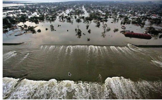
Levee failure in New Orleans following Hurricane Katrina (Feireiss 2009)
