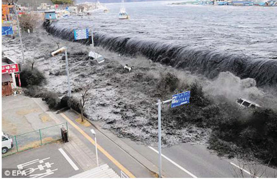
Levee failure in Japan during the recent tsunami (Zevenbergen 2011)
